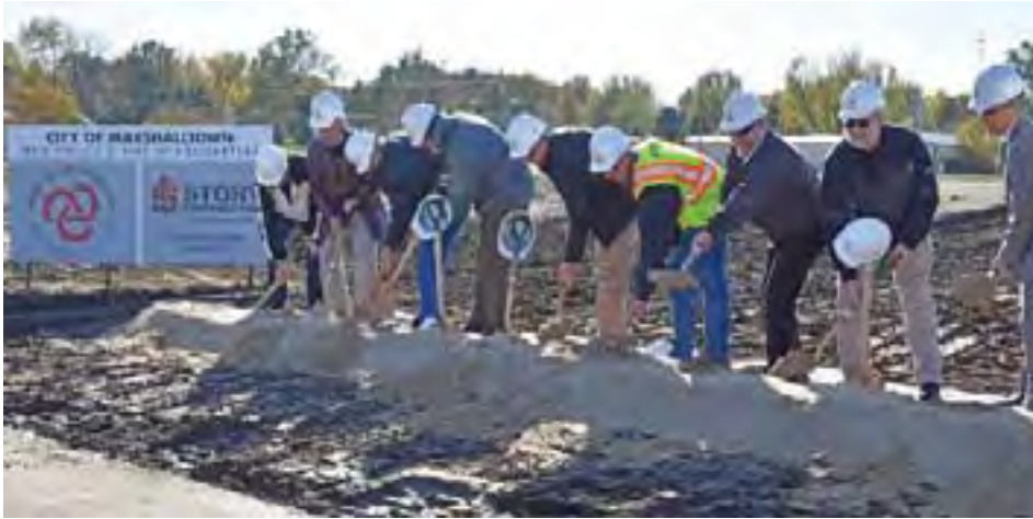
On October 24, Chamber Ambassadors attended the groundbreaking ceremony for the City of Marshalltown new Police & Fire Headquarters (900 block of South 2nd Street). Photo courtesy of the Times-Republican.
