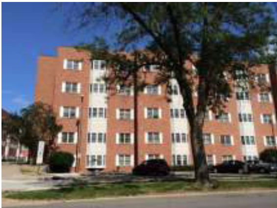
Older mid-rise senior apartments on north side (The Embers)
