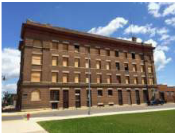
2. Senior LIHTC units under construction in former Iowa Wholesale building (downtown)
